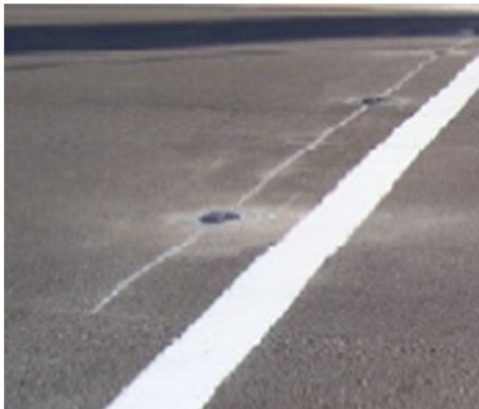
Fixtures Placed in Base Cans
