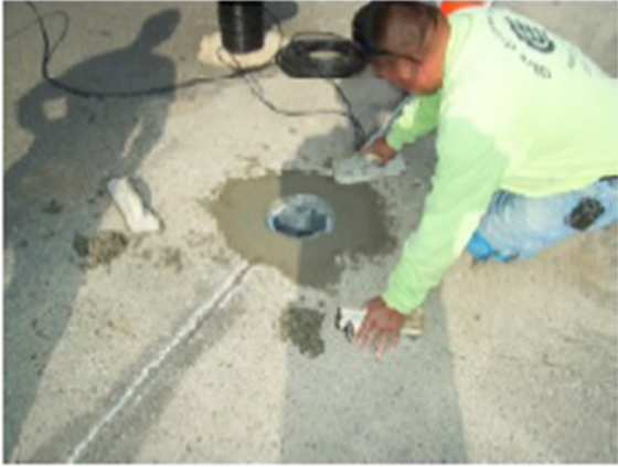
Base Can in Concrete
