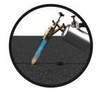
Dry the hole with a blowtorch to remove any moisture that may compromise the adhesion and effectiveness of the grout.
