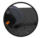
Using a disk cutter, open a connection between the holes with 1.2" (30 mm) width and 5.1" (130 mm) depth.
