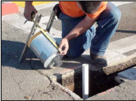
Mounting Jig Attached to Base Can
